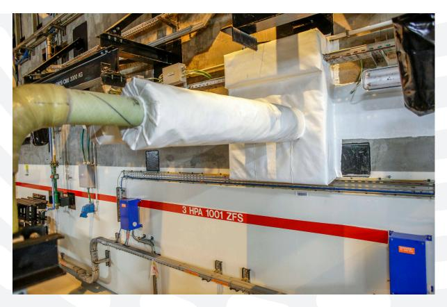
NuPLUG 5110 is a multicomponent firestop compound used to seal electrical, mechanical, blank and mixed feedthroughs, in walls and slabs
