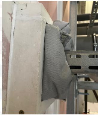
BagPART is an intumescent fireproof bag designed to seal cable passages in slabs, walls and drywall.
