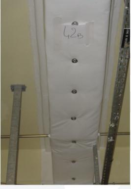
The NuSTRUCT 5110 is a flexible, fireproof, waterproof and airtight protection adaptable to all profiles. It is used as a fire protection on concrete structures in order to improve its fire resistance.
